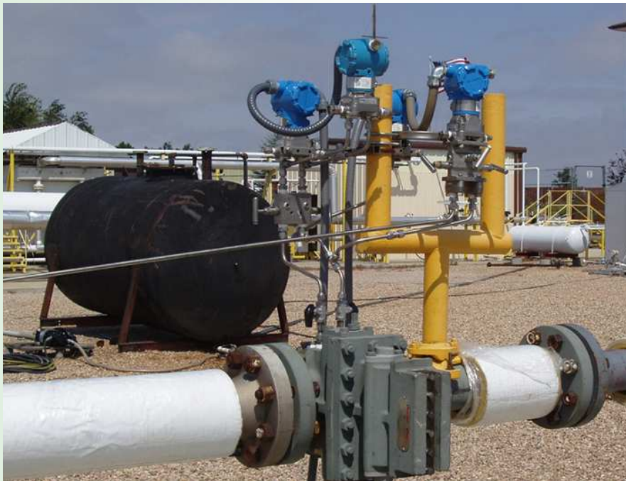
A Orifice Meter Installed with Diagnostics.
