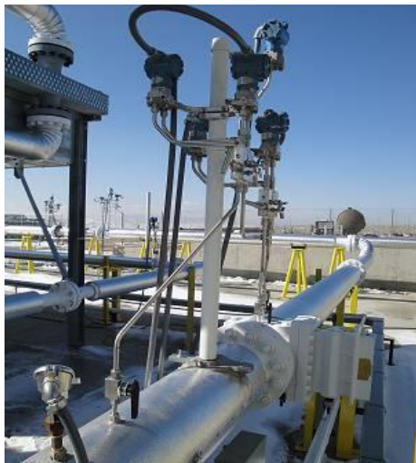
Fig 1. 8", 0.564 \beta Orifice Meter With Prognosis™.
